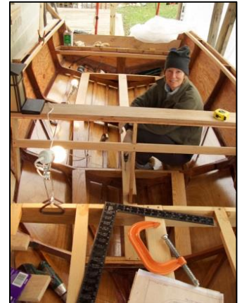
Installing the cockpit floors. (courtesy, Lisa Egeli)
